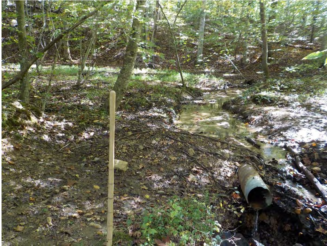
Photograph 3: Stream 3 crossing location (view SE), note existing CMP culvert
