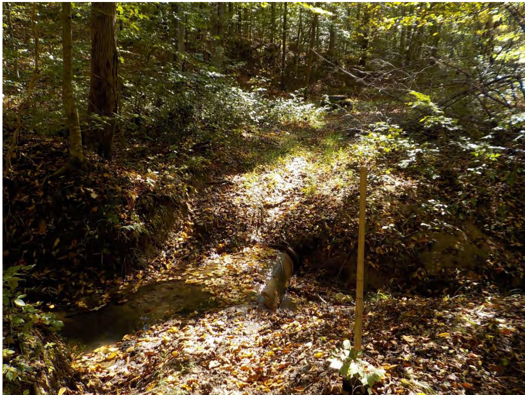
Photograph 4: Stream 4 crossing location (view S), note exposed sanitary sewer line
